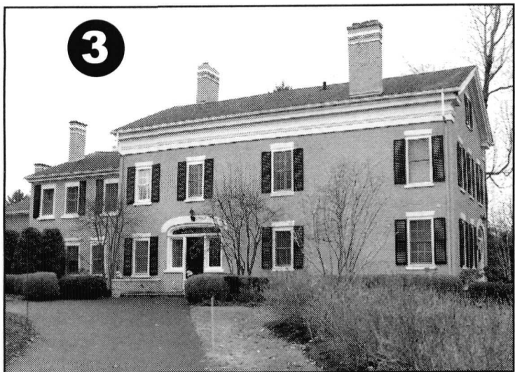
3 Babcock House - 1496 Clover Street, Brighton
